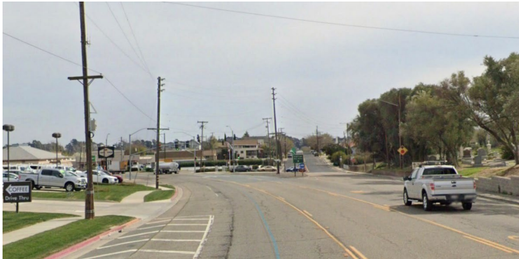
Existing Entrance to the City of Rio Vista on EB SR 12
