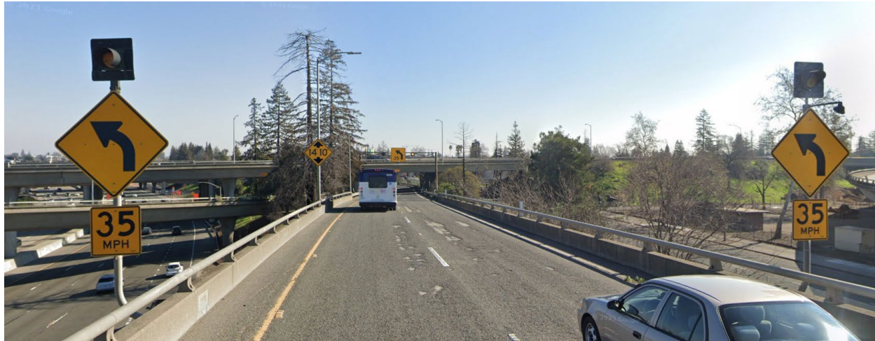
Flashing Beacons on US 50 EB to Business 80 Connector in Sacramento, CA (Google Maps)
