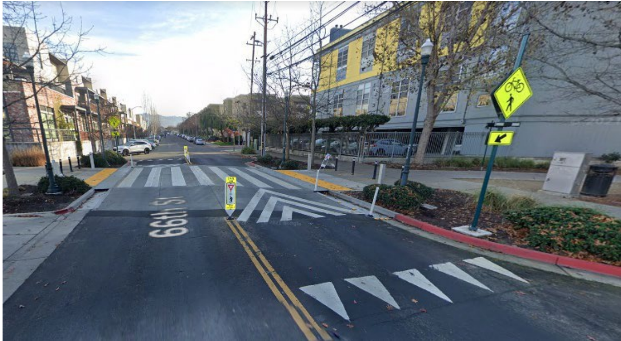
66 th St in Emeryville, CA (Google Maps)
