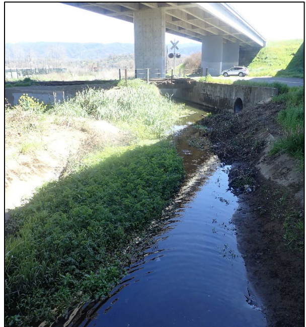
Photo 8. Looking downstream from box culvert at UK.21. In the background, a culvert that runs under Ford Road can be seen. Note the concrete lined slopes (April 4, 2023).
