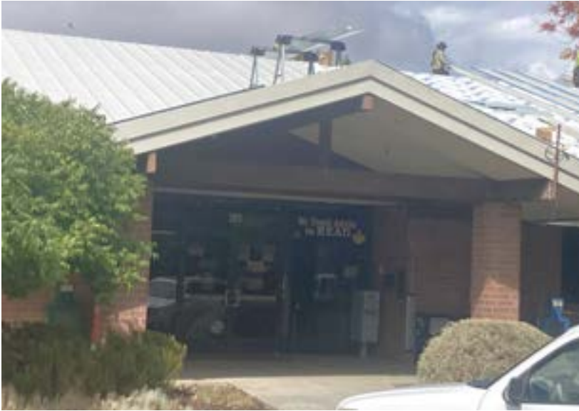
Willits roof construction.
