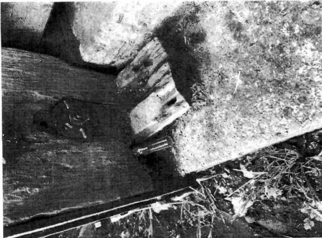
PLATE 3-SOUTH-EAST COLUMN WITH DECAY (3" SCREW DRIVER EMBEDDED)
