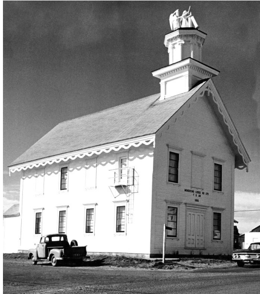
Masonic Hall (1866) at Lansing & Ukiah Streets
