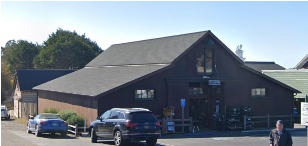
Mendocino Hardware Store with Composite Shingle Roof
