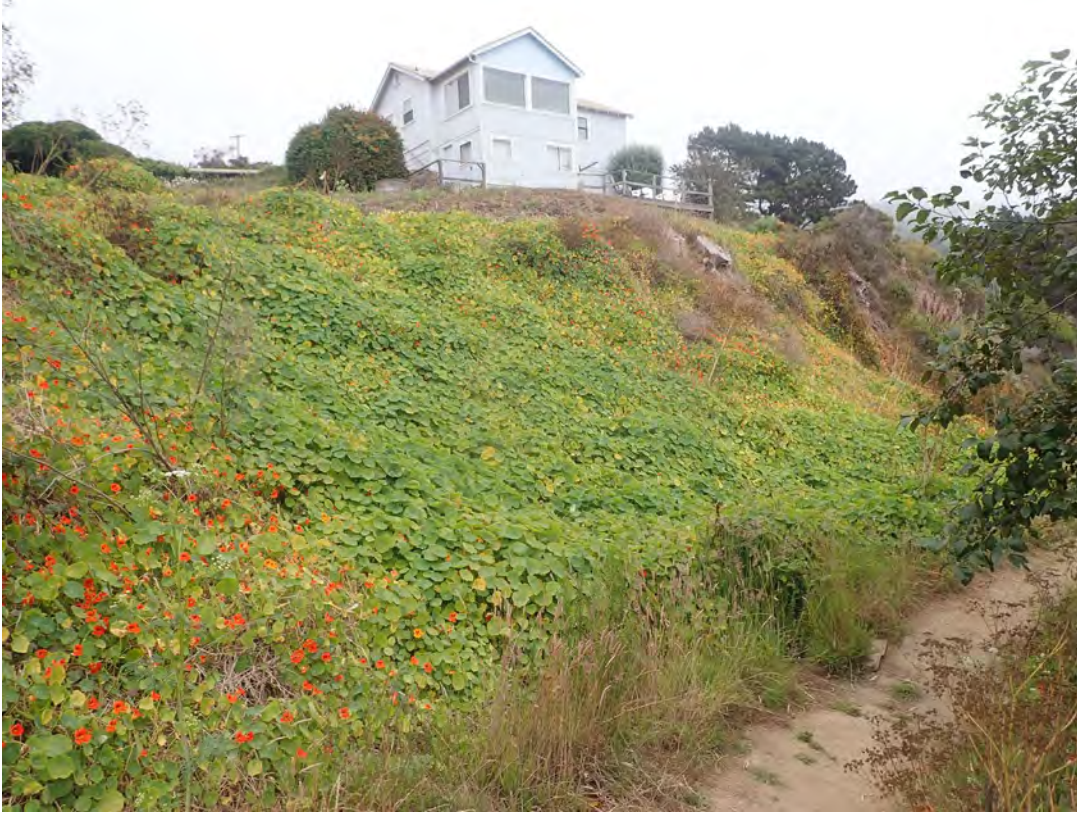
Figure 5. Non-native plants dominating eroding hillslope beneath residence.
