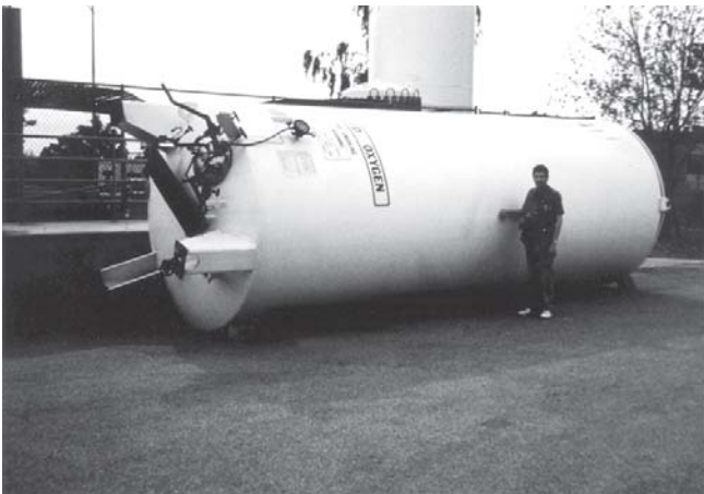
Figure 46 - The support pedestal system of this oxygen tank at Olive View Medical Center was damaged after the 1994 Northridge earthquake, leaving the tank leaning. The tank is shown after it was removed to allow for installation of a replacement unit.
