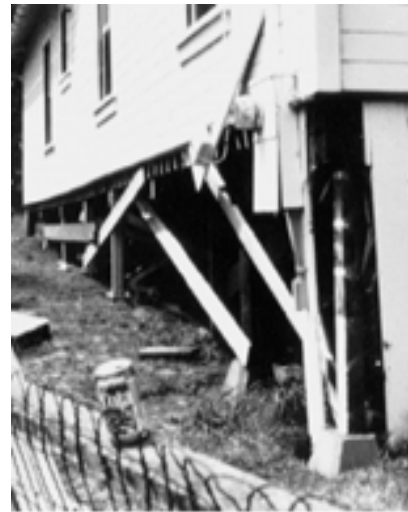
Figure 18 - The pier-and-post foundation under this home shifted during a recent earthquake.
