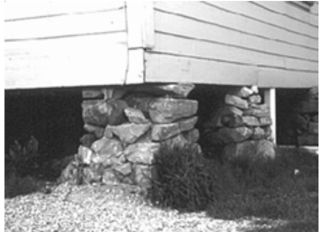
Figure 19 - This is an unreinforced stone foundation. They typically fail during earthquakes.
