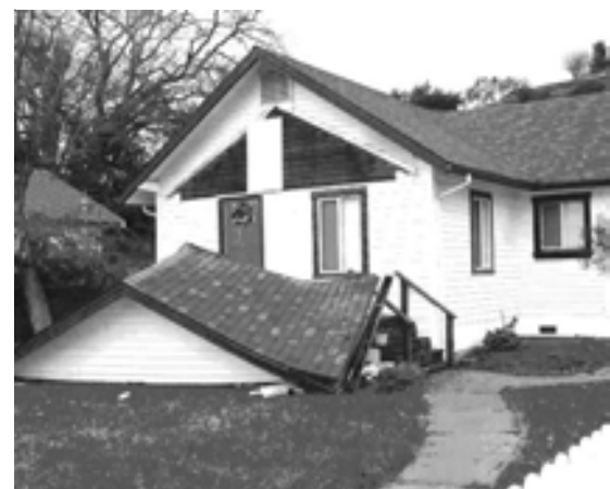
Figure 6 - San Simeon Earthquake, Dec. 22, 2003 The collapsed porch was not adequately attached to this single family residence.
