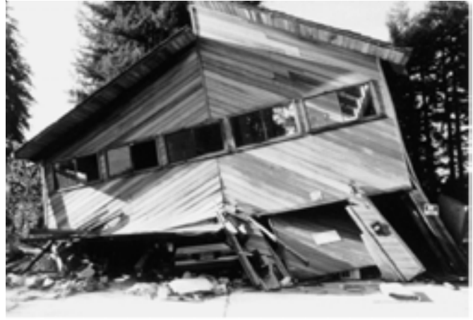
Figure 29 - This mountain home was built over a garage, and its walls were not strong enough to withstand an earthquake.
