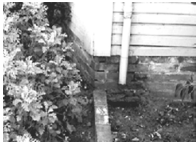
Figure 20 - Note the bricks exposed in this unreinforced masonry foundation.
