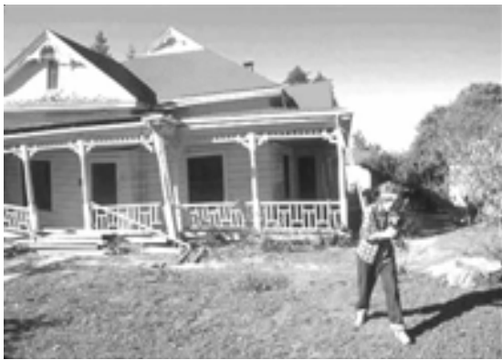
Figure 2 - Loma Prieta Earthquake, Oct. 17, 1989 Home moved off of its foundation and was considered a total loss.
