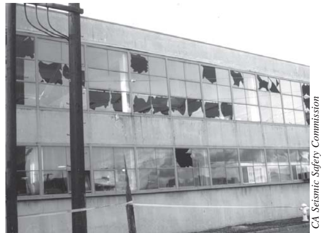
Figure 56 —The windows in this San Francisco building probably broke because its frame flexed too much in the Loma Prieta earthquake of 1989.
