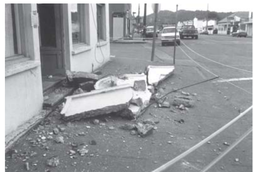
Figure 20 - Unbraced Parapets can Injure and Kill - This parapet on the front of the building in Figure 18 fell on the sidewalk.
