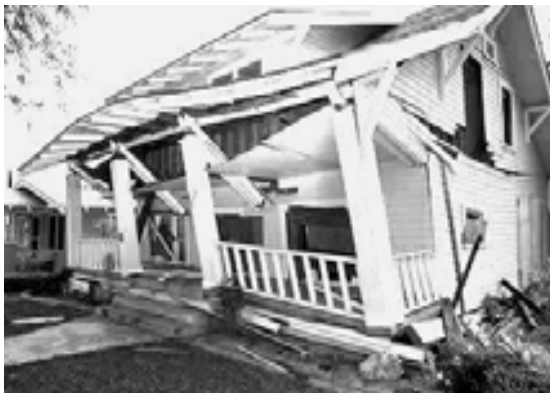
Figure 3 - Northridge Earthquake, Jan. 17, 1994 Single family residence damaged due to failure of multiple elements.
