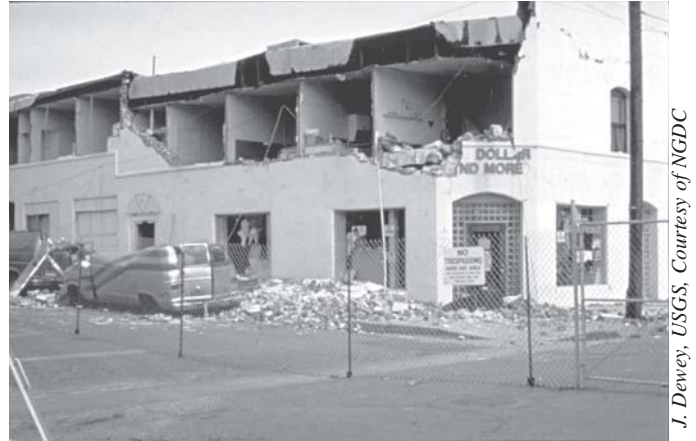
Figure 16 - The second-story wall of this unreinforced masonry building was not well-tied to the roof, and the building collapsed during the 1994 Northridge earthquake.
