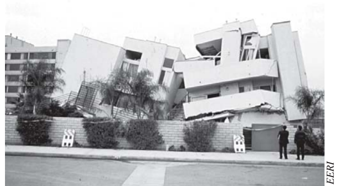
Figure 32 —This modern wood-frame apartment building had a central driveway. It collapsed inward over unbraced entrances to crush first-story parking during the 1994 Northridge earthquake.
