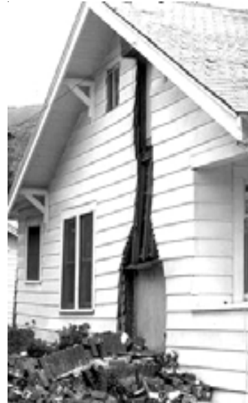
Figure 4 - Northridge Earthquake, Jan. 17, 1994 Chimney Collapse - common type of damage to unreinforced masonry.
