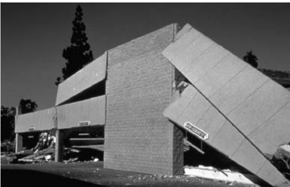
Figure 5 - Concrete Parking Structure Collapse.
