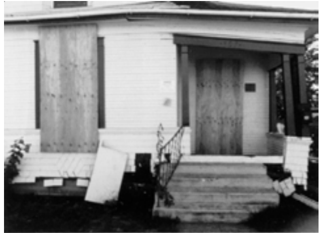
Figure 13 - This home wasn't bolted and slid off its foundation. Sometimes the damage can be so bad that houses have to be demolished.
