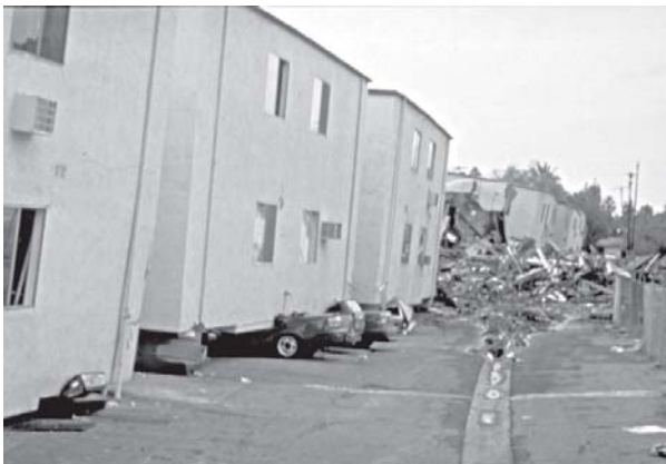
Figure 31 —A similar apartment building's soft story collapsed on cars during the same earthquake.
