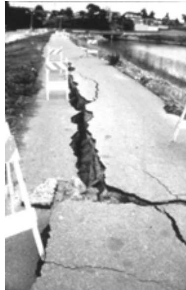
Figure 39 - Lateral Spreading. Loma Prieta Earthquake, October 17, 1989. Lateral spreading damage levee road along the San Lorenzo River.
