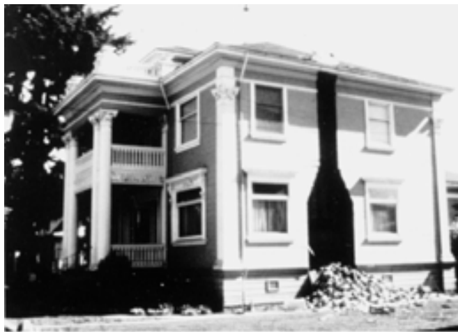
Figure 33 - This unreinforced chimney fell during a recent earthquake.
