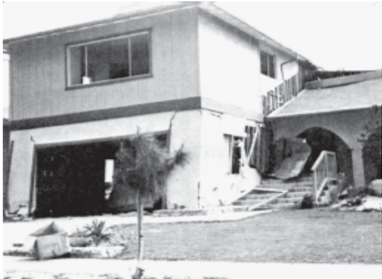
Figure 1 - San Fernando Earthquake, Feb. 9, 1971 Severely damaged split level 1 and 2 story wood frame dwelling. The one story portion dropped about 3 feet.
