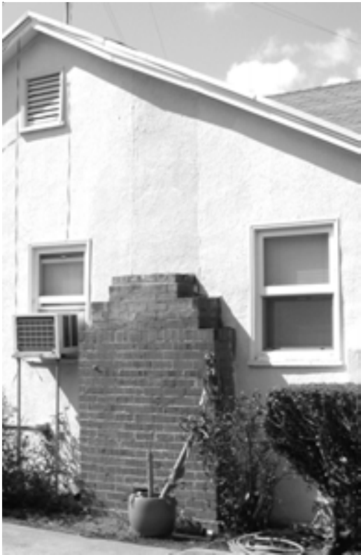
Figure 35 - Photo showing damaged chimney removed. Note that the fireplace is now not functional.
