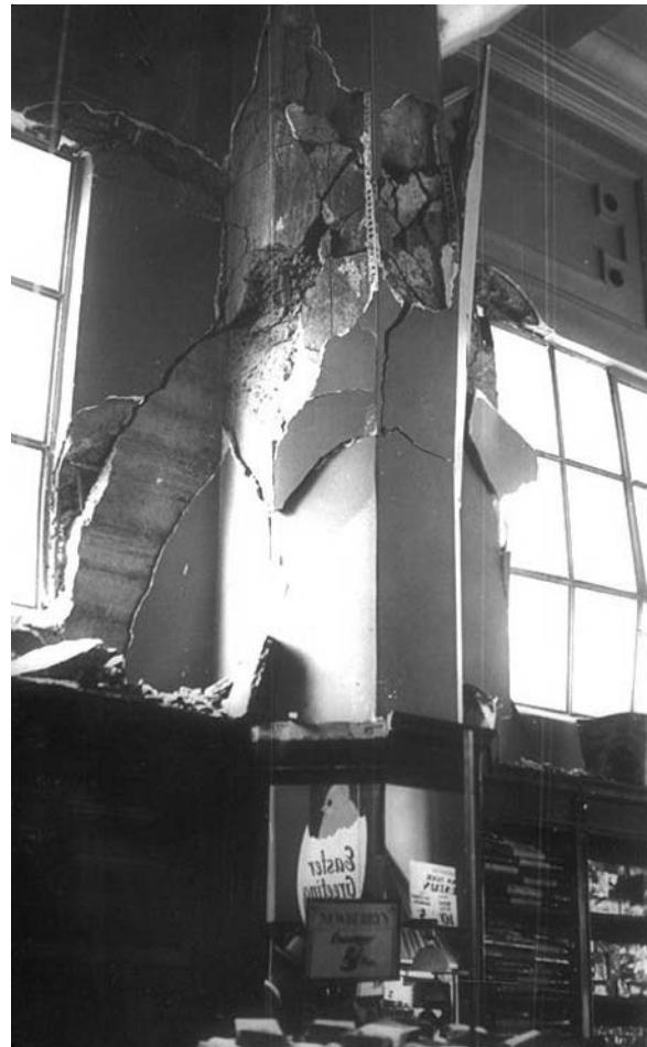
Figure 34 - This unusual building with a tall story, long spans and large windows was severely damaged in the 1933 Long Beach Earthquake.
