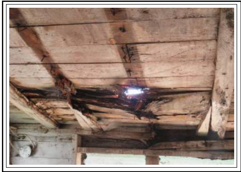
Additional ceiling detail - note daylight
