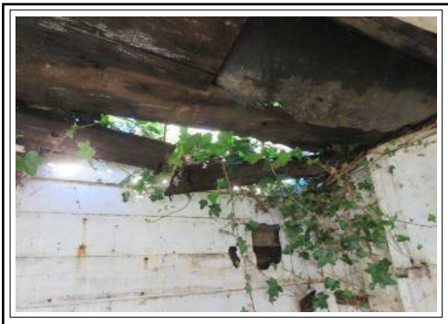
Caved in roof structure in former residence.
