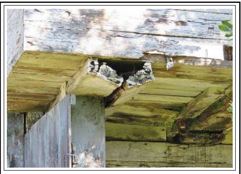
Building detail - note rot and damaged framing member on detached structure.
