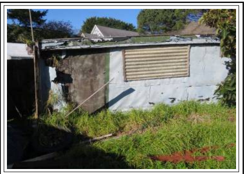
Former garage - deteriorated beyond repair
