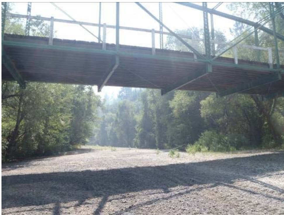
Photo 2 - View of Existing Bridge from Mill Creek Channel, facing south
