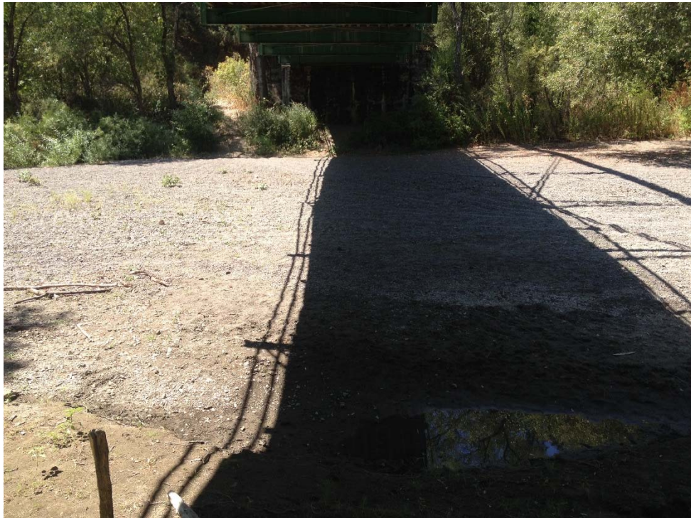
Photo 10 - View of stream channel, facing west.
