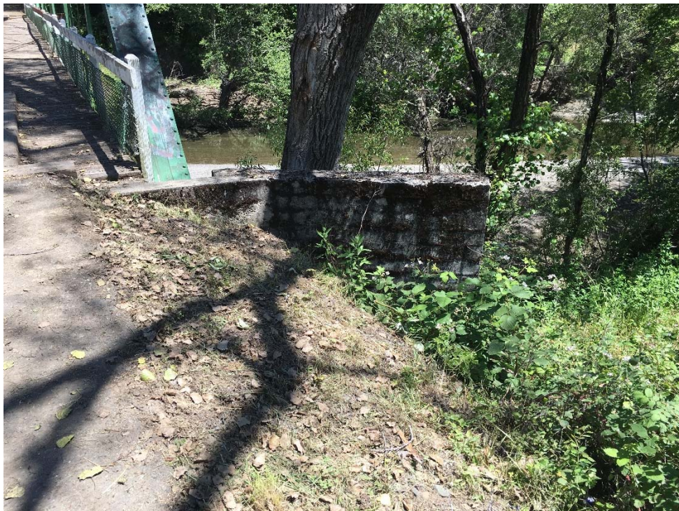
Photo 12 - View of bridge abutment, facing southeast.
