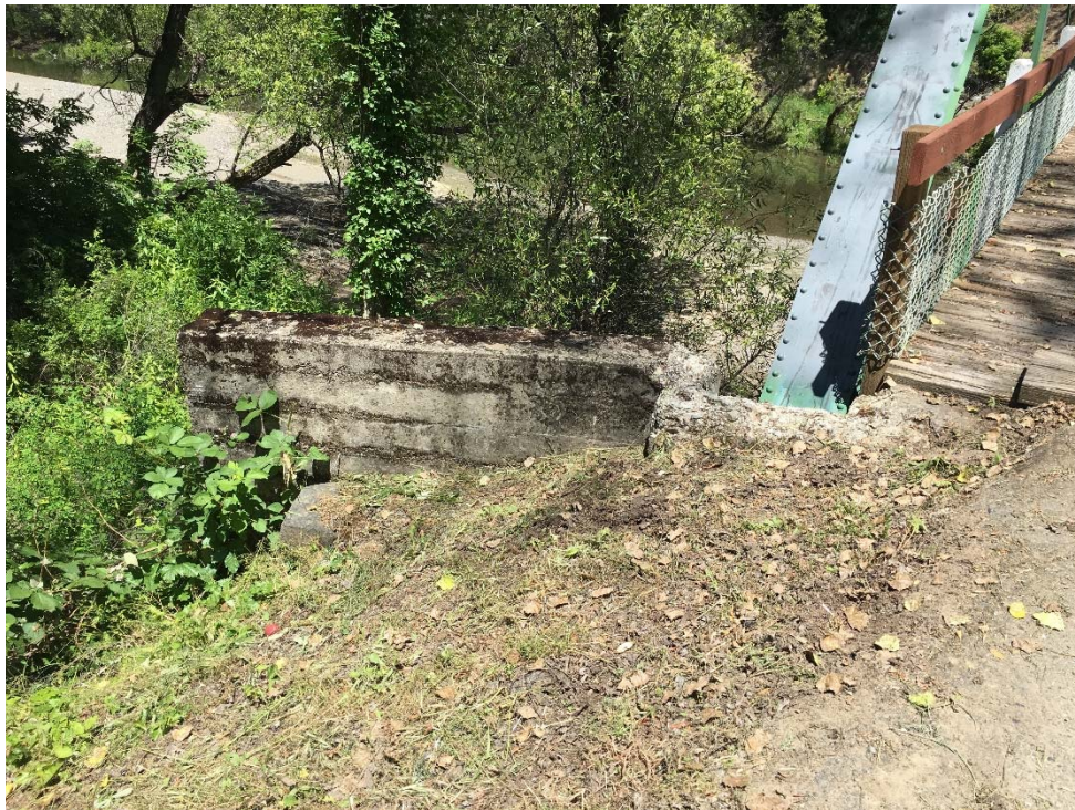
Photo 11- View of bridge abutment, facing northeast.
