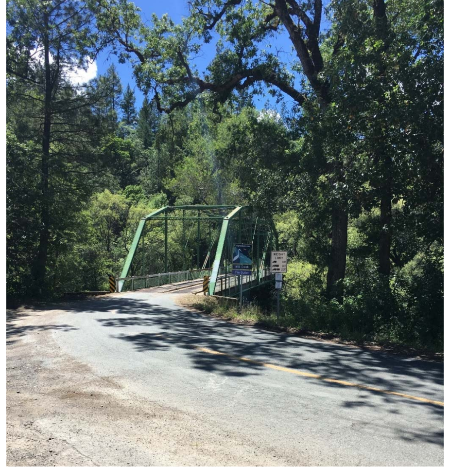
Photo 6: View of bridge approach, facing east.
