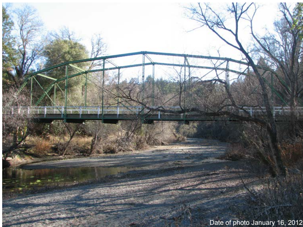
View of bridge and creek looking south.
