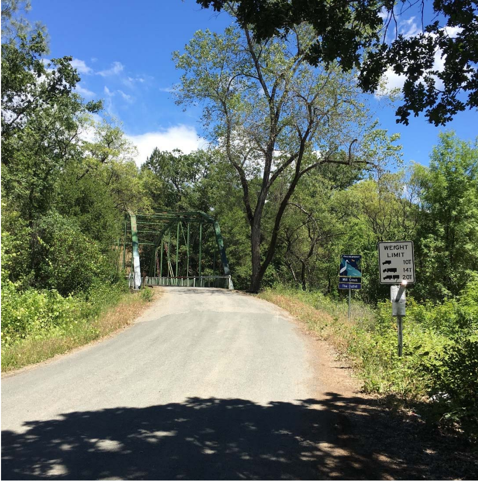
Photo 5: View of bridge approach, facing west.
