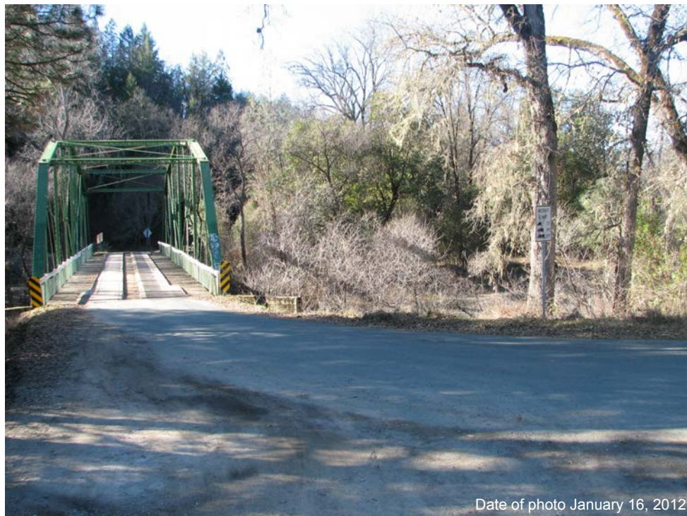
View of bridge and roadway approach looking west.
