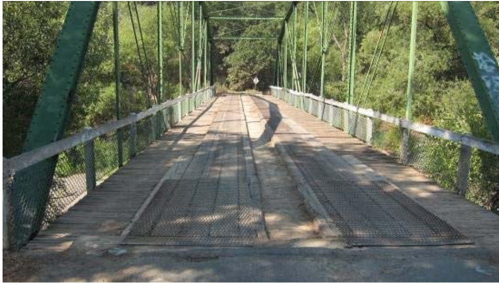
Photo 1 - View of Existing Bridge Deck, facing west
