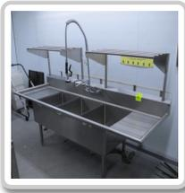
**3-compartment sink w/ L & R drainboards, prewash spray & overhead drying racks**
