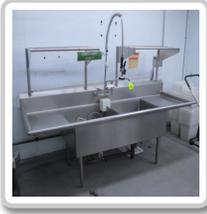
**2-compartment sink w/ L & R drainboards, prewash spray & overhead drying racks**
