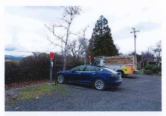
Plate 19 Tesla Level 2 charger at the Terra Savia Winery in Hopland
