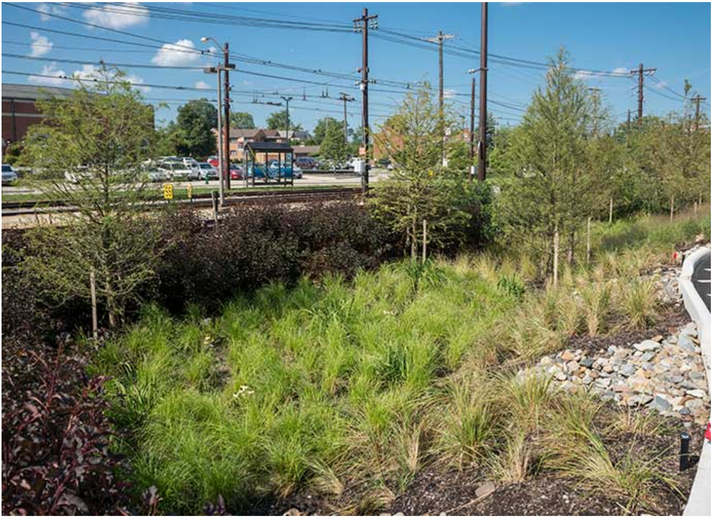
The bioswale off the rear parking lot of the Upstairs apartments
