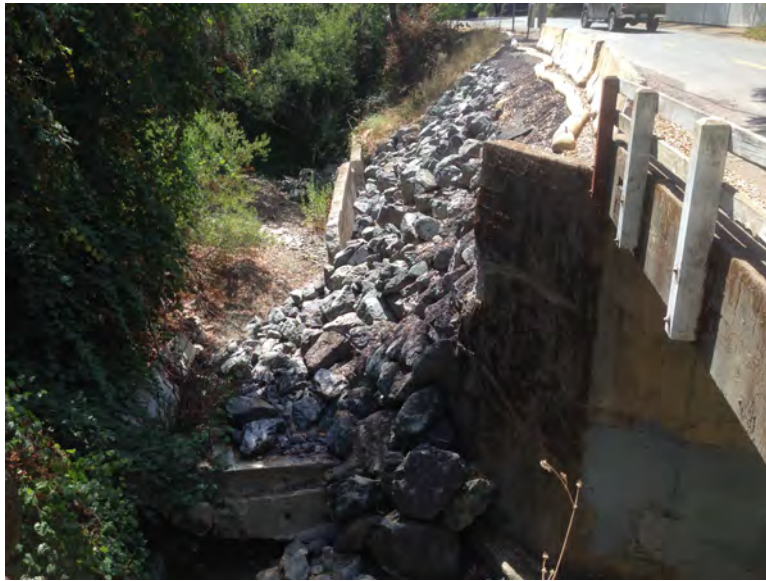
Photo 3. Failed retaining wall, painted guard rail, wing wall, grey paint covering graffiti, 8/26/15
