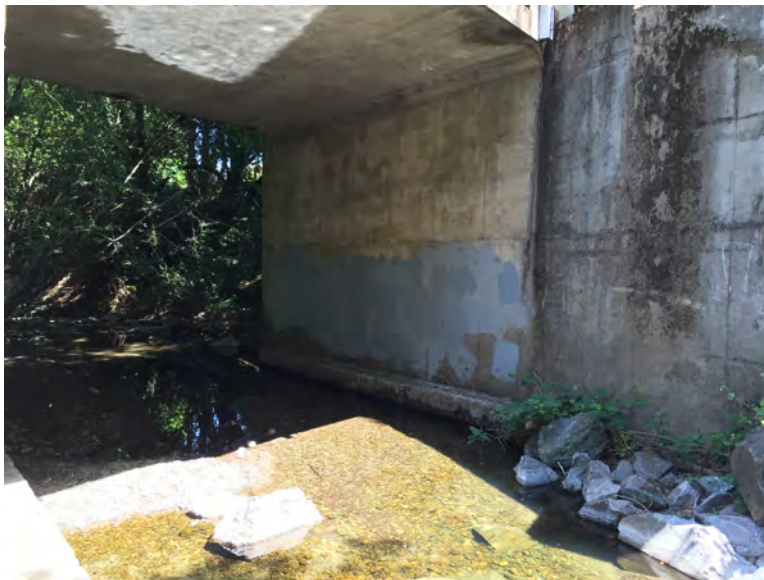
Photo 8. Paint on pier walls, two coats, both sides of bridge, covering graffiti, 5/11/16
