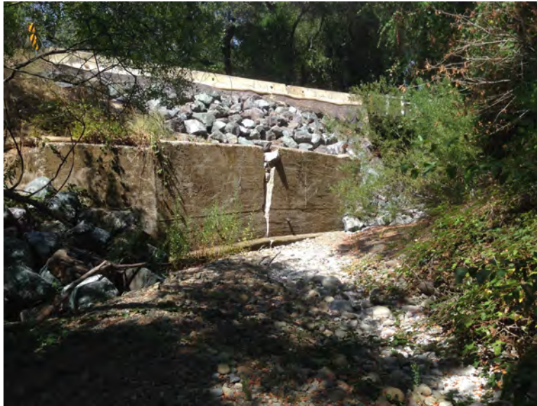
Photo 5. Cracked retaining wall upstream of bridge on west bank, 5/11/16
