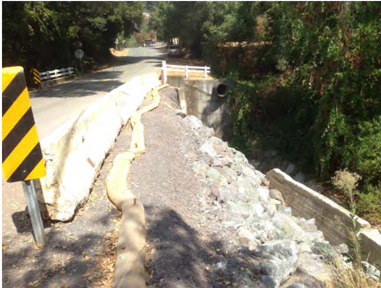
Photo 1. Project Site. Failed retaining wall, rock slope protection, shotgun storm drain, 8/26/15
