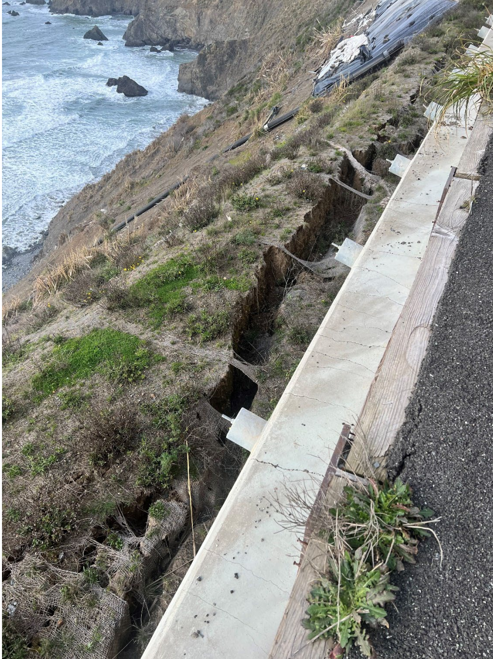
Photo taken 3/5/25 showing stress cracks in newly installed whaler
