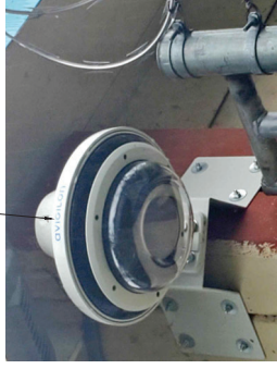
EXISTING 270-DEGREE SECURITY CAMERA NO SCALE
