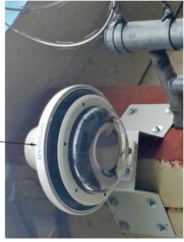
EXISTING 270-DEGREE SECURITY CAMERA NO SCALE
