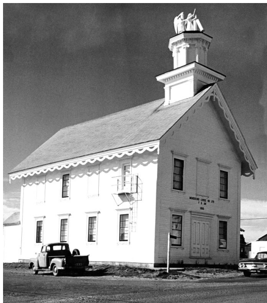
Masonic Hall (1866) at Lansing & Ukiah Streets
